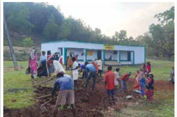
School Ground repairing under DFW Programme
